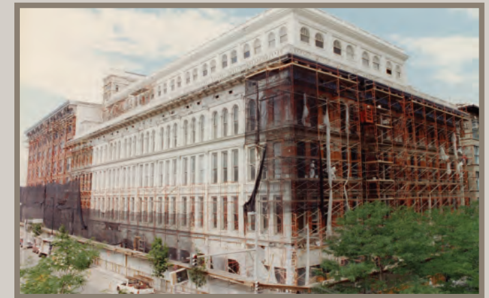
Preservation of the historic Denver Dry Building at 16th and California Streets incorporated significant exterior renovation, including removal of more than 30 layers of lead-based white paint to expose the red-brick, sandstone, and limestone surface of the original building.
