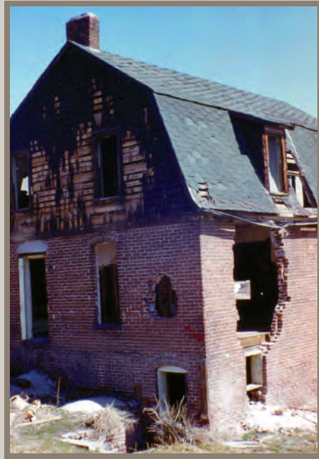
Residential properties in the Avondale neighborhood in the 1950s were interspersed among junkyards, taverns, warehouses, and factories. Many, like this home at 1329 Hazel Court, were eventually abandoned and fell victim to structural scavenging.
