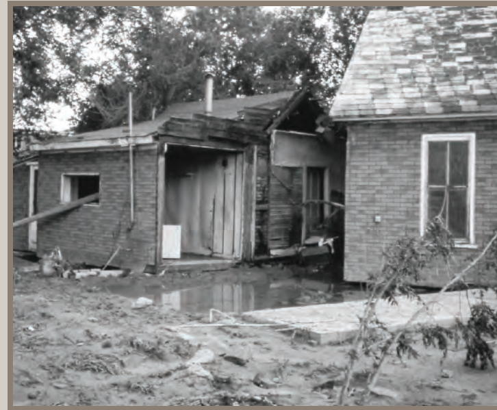
This house was washed off its foundation by the flood of 1965, which devastated the Jerome Park neighborhood. DURA improvements to the area included a new 42" storm sewer line that enabled redevelopment of the area into a successful commercial-industrial zone immediately east of Interstate 25.
